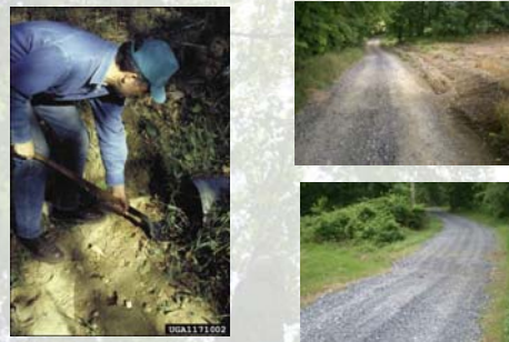
Cleaning out culverts
